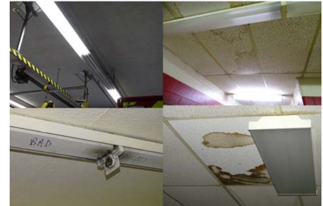
Central Fire Ceiling and Lighting
